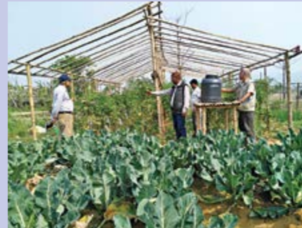
Plastic House under construction
