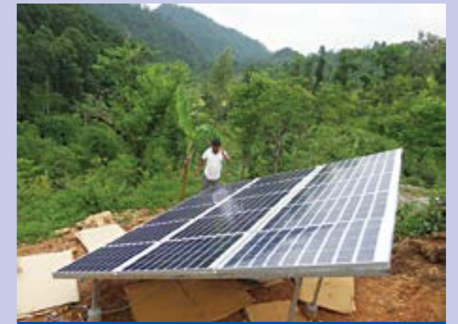
Installation of Solar Panel for Lift Irrigation at Saune
